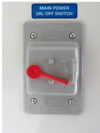
**Figure 4-1: External PSE ON/OFF Switch in the OFF position**
