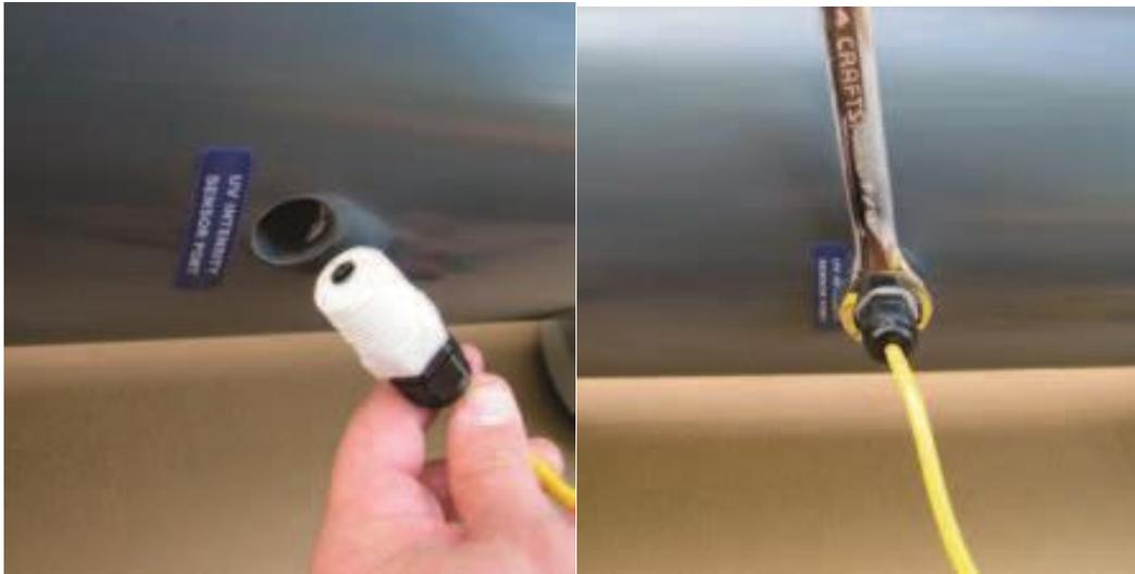
**Figure 2-9: UV Intensity Sensor Location**
